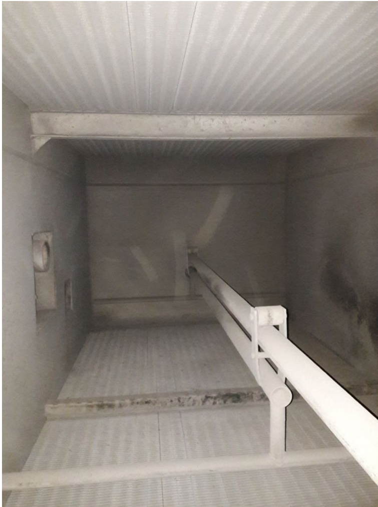
EG10XL discharge nozzle cleaning right side of finned tube ECO bundles. Rake soot blower stays installed.
