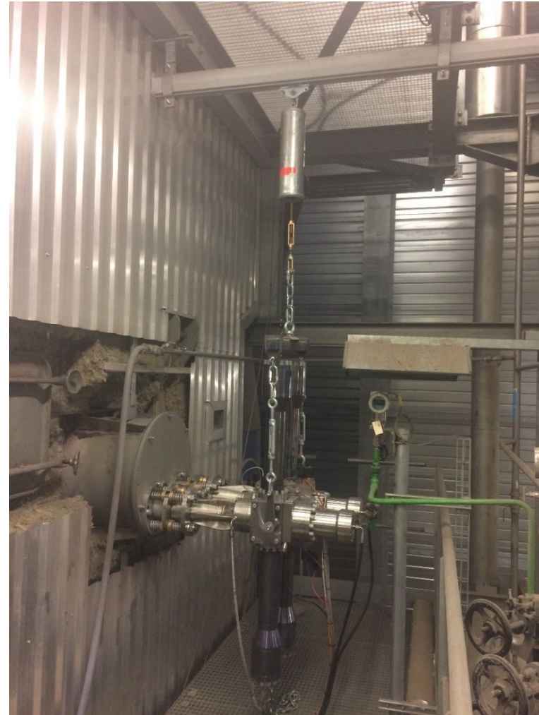
TwinL 90° rotated cleaning left side of finned tube ECO bundles. Met tight installation restrictions outside of boiler.
